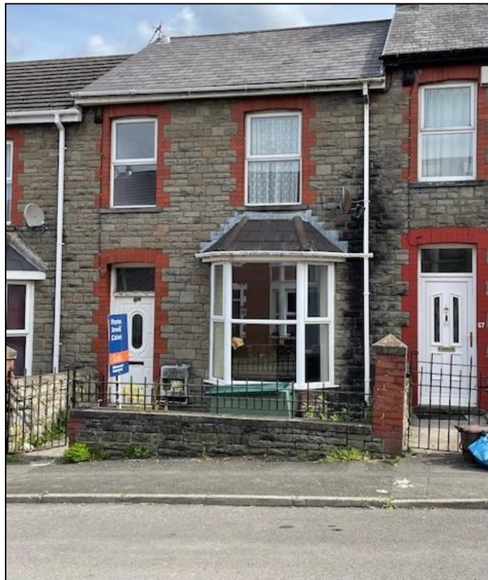
Figure 6 Photo of Front Elevation of Property
