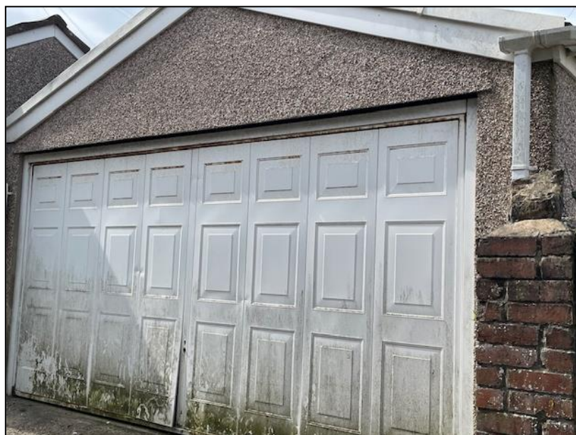
Figure 7 Photo of Rear Elevation of Property
